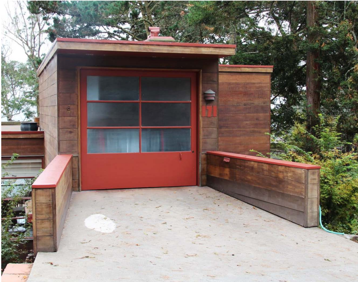
Above: View looking south towards the street-facing facade level with the sidewalk (2015).
